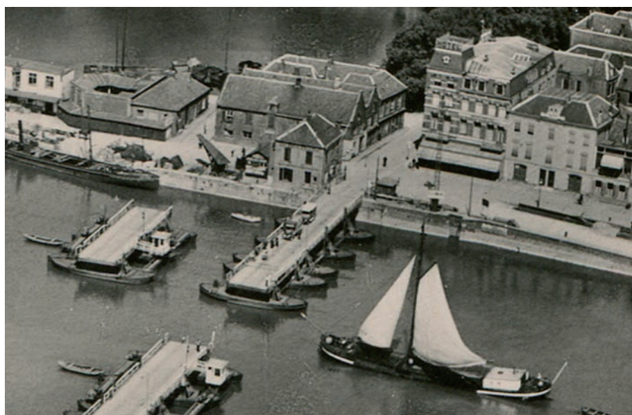
Point of interest 18: A pontoon bridge
